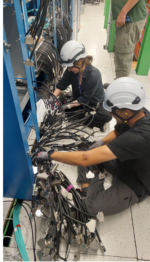
Figure 8: Cabling Work Underground in ATLAS
